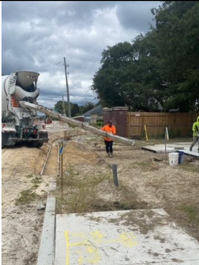
Formed and poured Driveway curb and gutter
