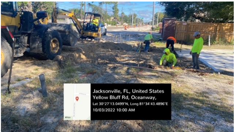
Formed and poured Driveway curb and gutter
