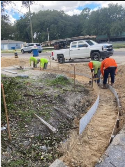
Formed and poured Driveway curb and gutter
